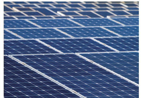
Solar Array Load Testing
